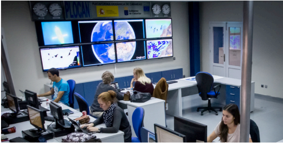
Illustration 9. Operation control room
