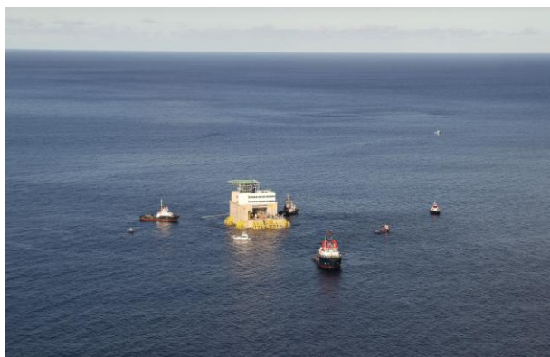
Illustration 20. Photo of the mooring operation
