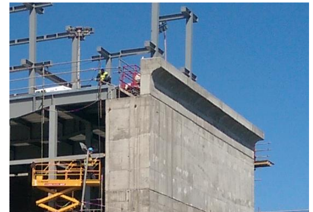
Illustration 4. Close-up of the construction of the breakwater at 17.8 m above sea-level
