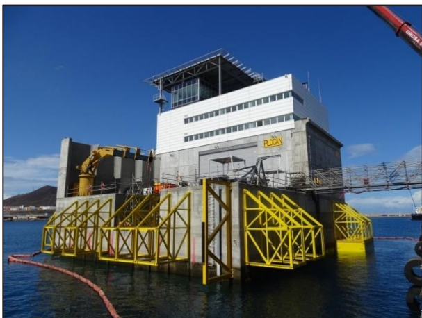
Illustration 18. Fitting the stabiliser structure
