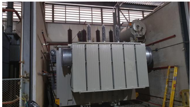
Figure 10. Supply and installation of the power transformer in the Jinámar power station
