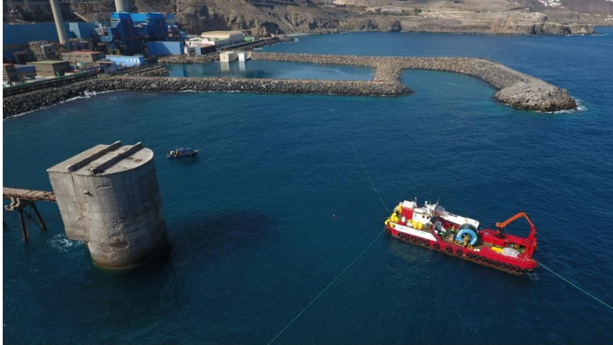
Figure 4. Mooring the cable-layer to start installation operations
