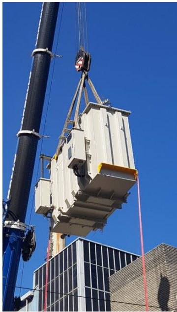
Figure 10. Supply and installation of the power transformer in the Jinámar power station
