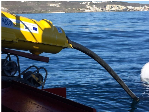
Figure 5. Laying the splice
