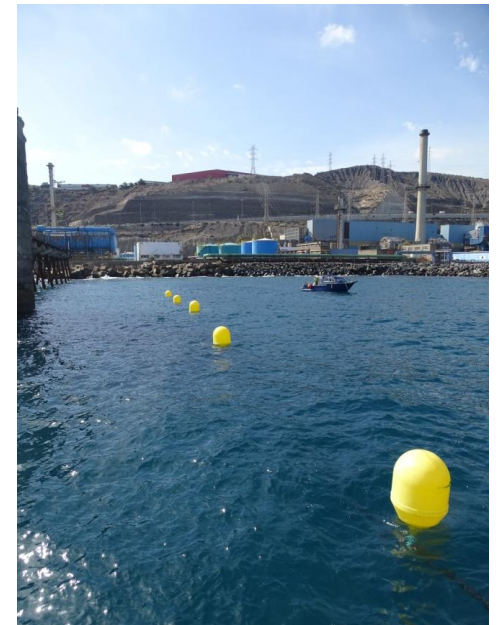
Figure 7. Start of the splicing operation
